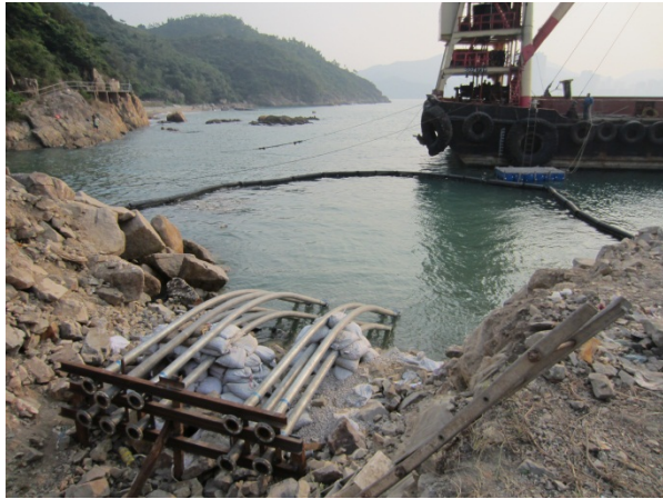
Photo 1 - A silt curtain was employed around the seawall area.
