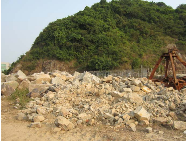
Photo 3 - Tarpaulin sheets to cover dusty stockpiles to prevent dust generation were absent from the construction site.
