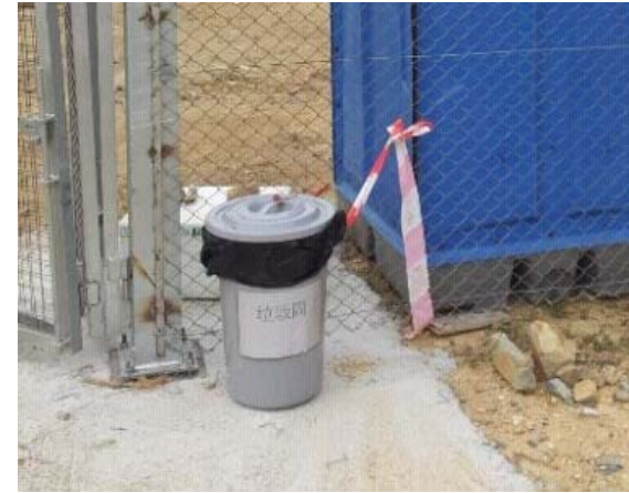
Photo 2 - A rubbish bin was placed on site in the next day of site inspection.
